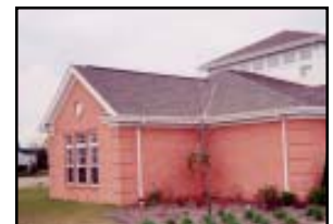
BUILDING END FACADE
