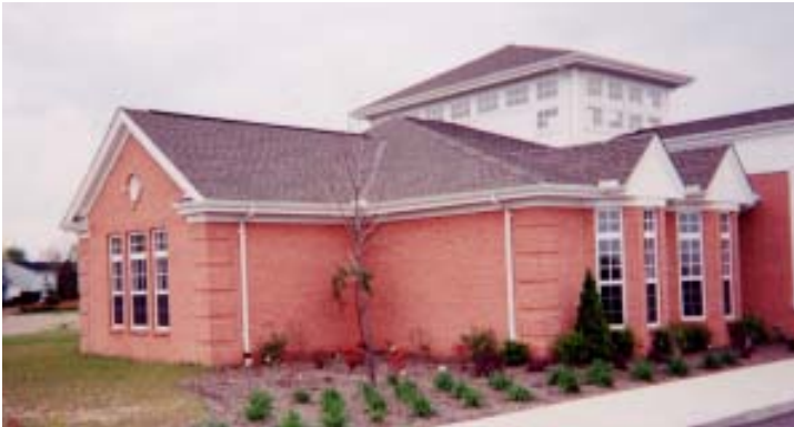
BUILDING END FACADE
